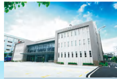
LESSO Research Institute & Testing Center
